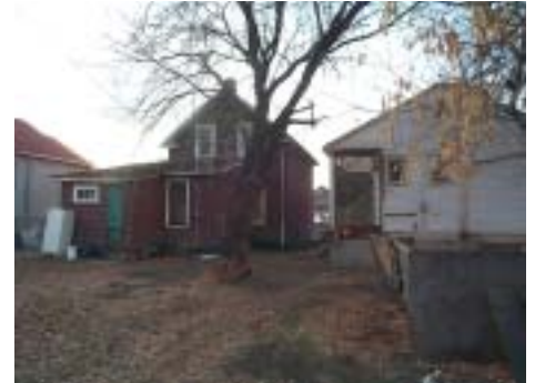
Houses to be razed for new family units. Run-down, unsafe, and very energy inefficient, houses like these rent for $700/month plus utilities. A cold snap in winter pushes the monthly costs to over $1000/month.
